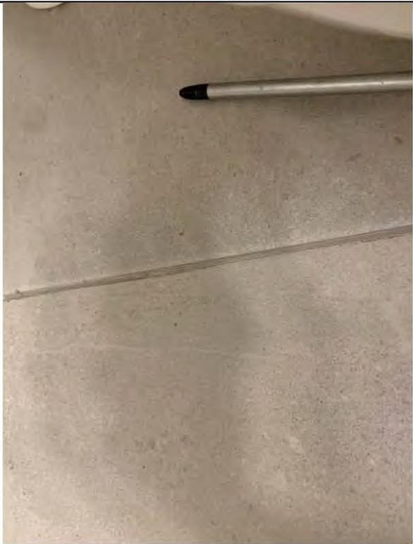
A close-up photograph of a light-colored floor tile joint, similar to the one in the first photo. A silver pen with a black tip is placed horizontally across the joint. The joint appears slightly recessed or uneven. | <p>Фото №29.<br/>Пустоты при<br/>простукивании напольной<br/>плитки на кухне</p> |
